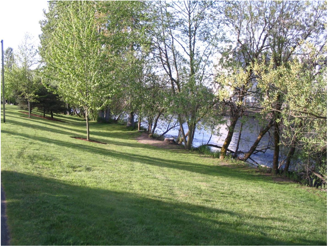
Photo 2. View looking upstream towards Logan Avenue of the I-type Floodwall on the left bank of the Cedar River with Renton Airport to the right (West).
